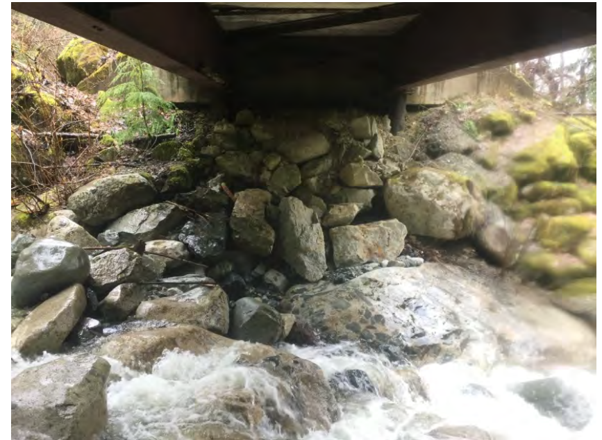
Left Bank Abutment when facing downstream
